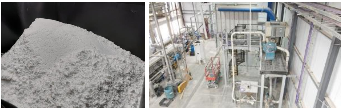
Figures 1-2. Rincon Lithium Project – 2,000tpa Operation Commissioning Works
