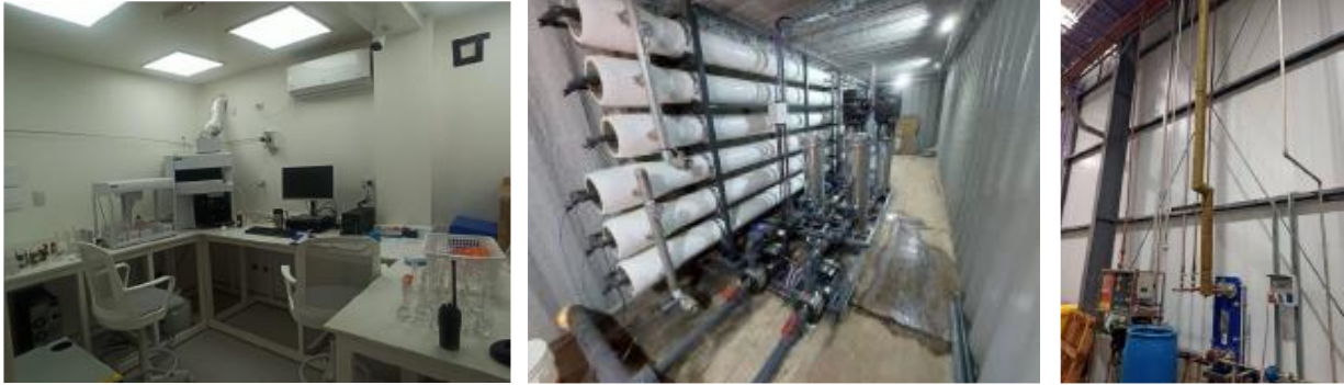
Figures 4-6. Rincon Lithium Project – 2,000tpa Operation Commissioning Works
