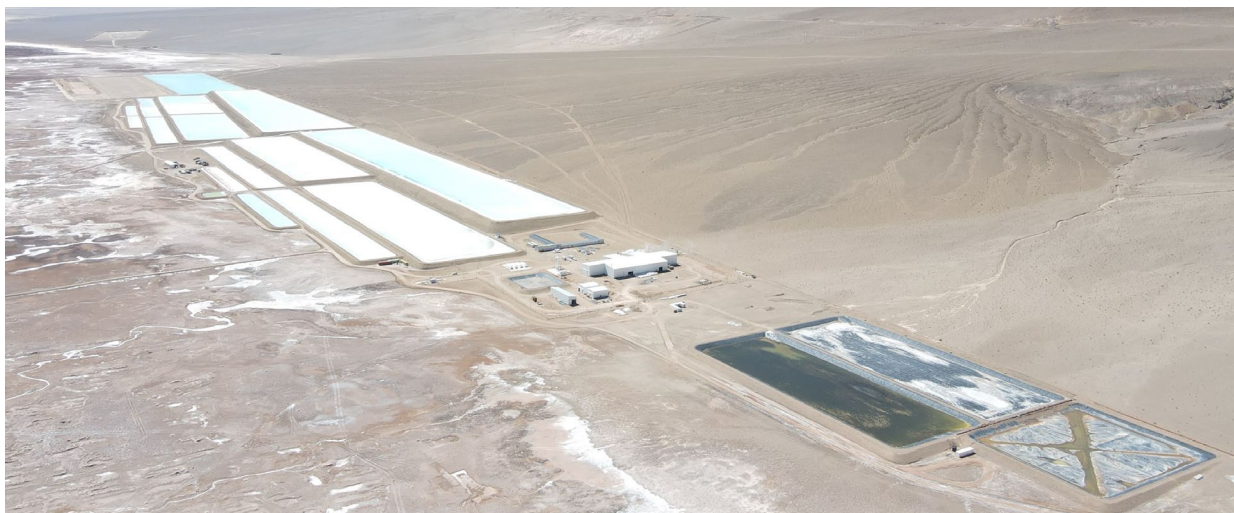
Figure 2. Rincon Lithium Project – 2,000tpa Operation
