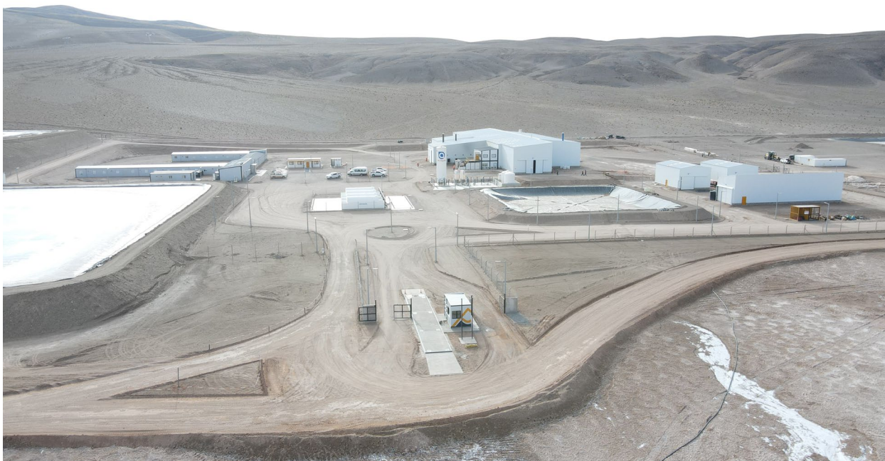
Figure 1. Rincon Lithium Project – 2,000tpa Operation
