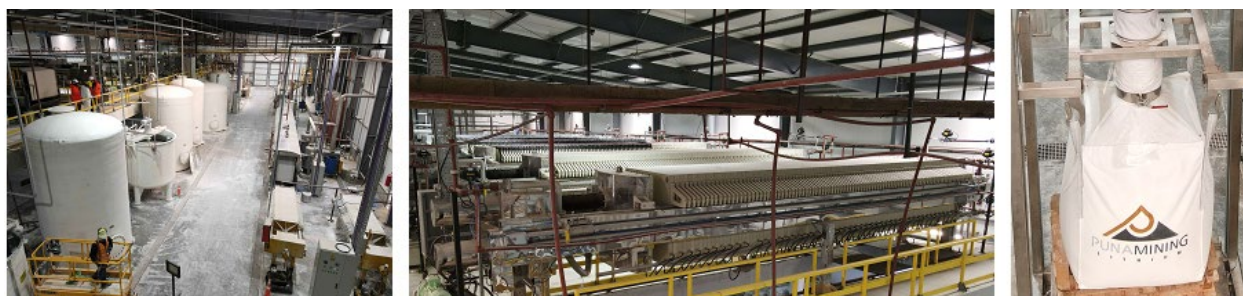
Figures 2-4. Rincon Lithium Project – 2,000tpa Operations
