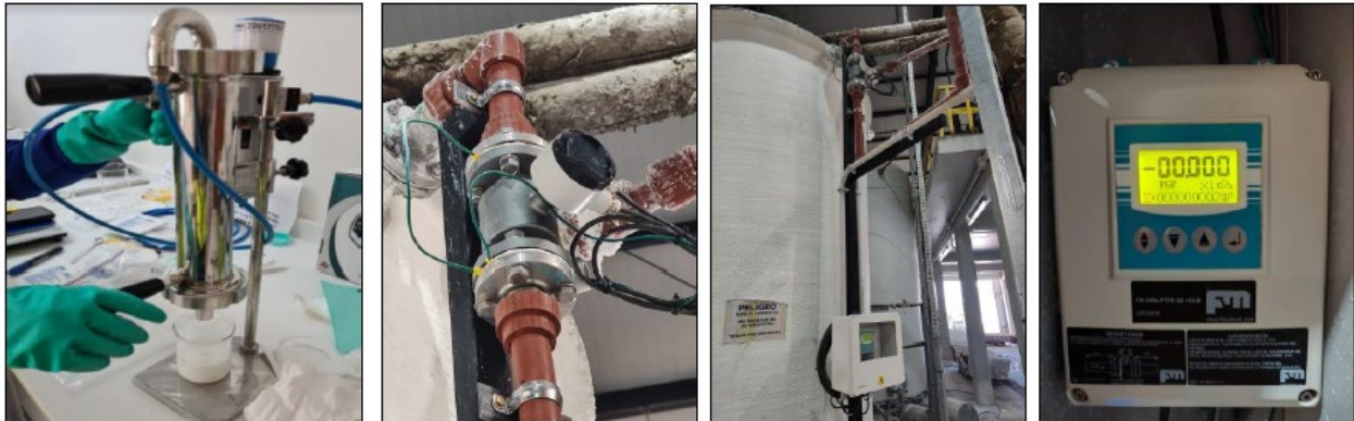
Figure 2. Rincon Lithium Project – 2,000tpa Operational Works
