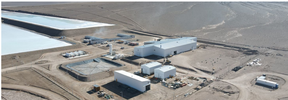
Figure 2. Rincon Lithium Project – 2,000tpa Operational Works
