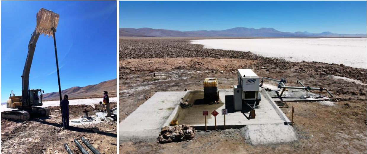
Figures 1-2. Rincon Lithium Project – New Brine Pump Installation Works
