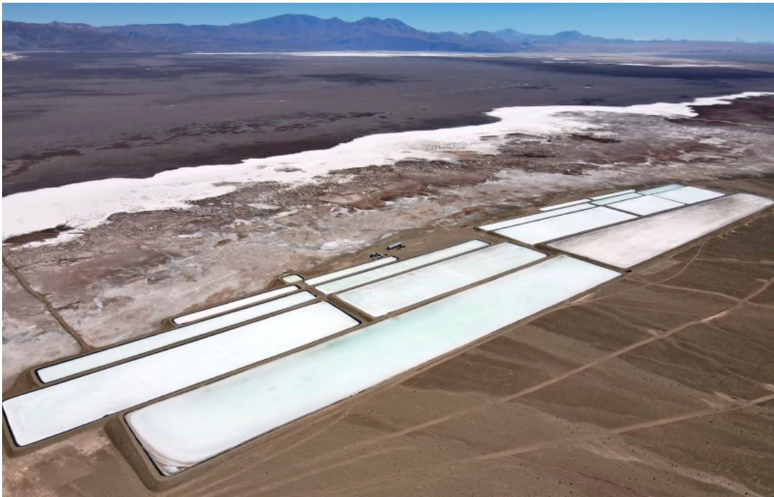
Figure 3. Rincon Lithium Project – 38Ha Operational Evaporation Ponds
