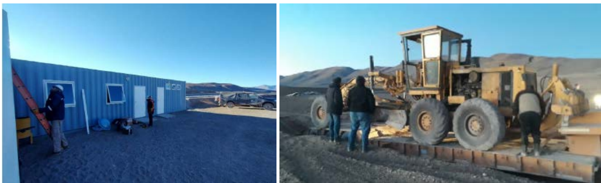
Figures 1-2. Rincon Lithium Project – 2,000tpa Operation Site Works in Progress
