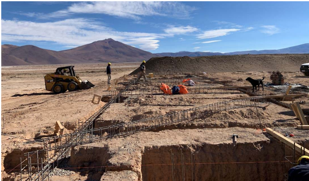
Figure 3. Rincon Lithium Project – 2,000tpa Operation Site Works in Progress
