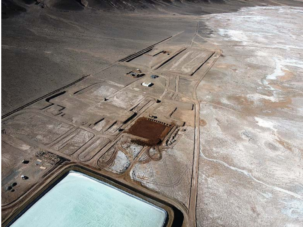
Figure 2. Rincon Lithium Project – 2,000tpa Operation Site Works in Progress
