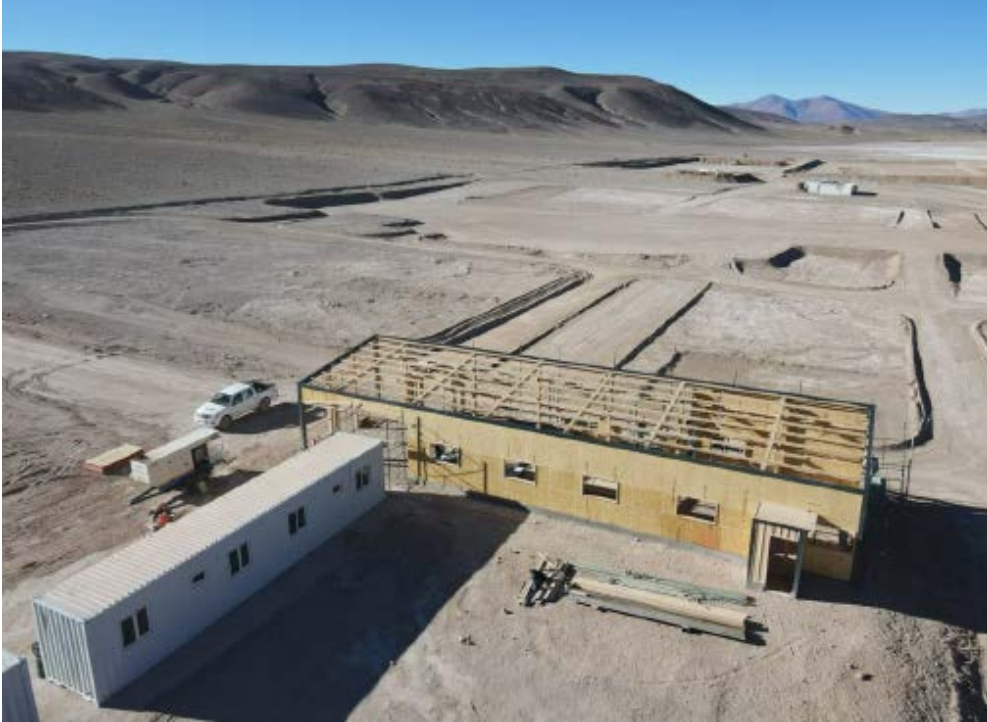
Figure 1. Rincon Lithium Project – 2,000tpa Operation Site Works in Progress
