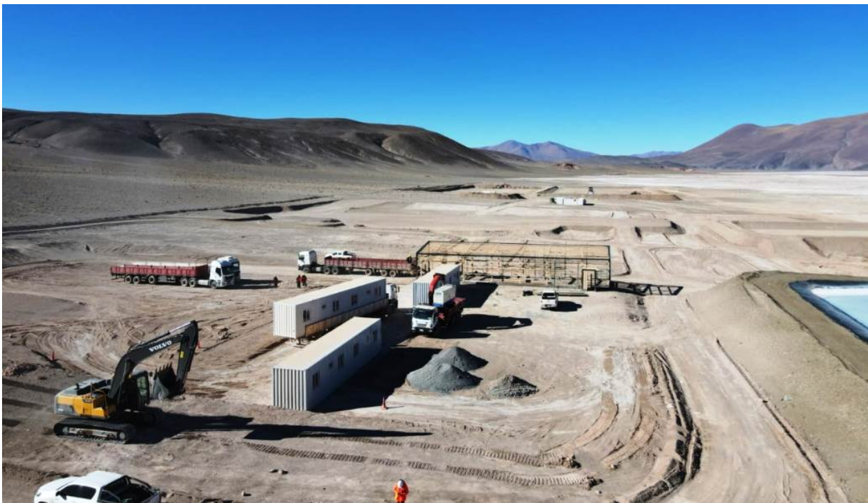
Figure 4. Rincon Lithium Project – 2,000tpa Operation Works in Progress (camp construction works)
