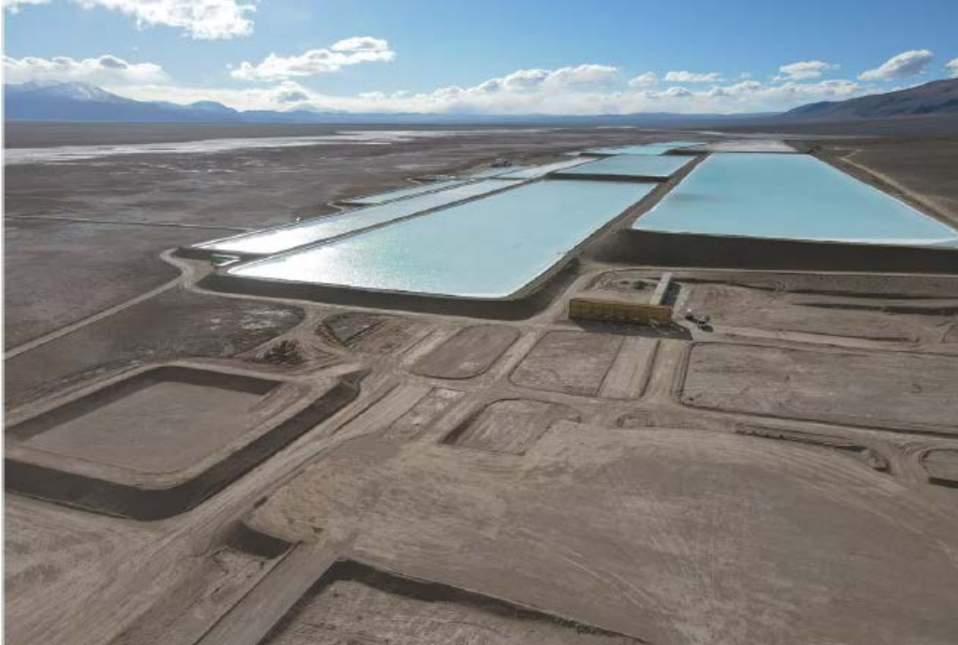
Figure 5. Rincon Lithium Project – 2,000tpa Operation Site Works in Progress
