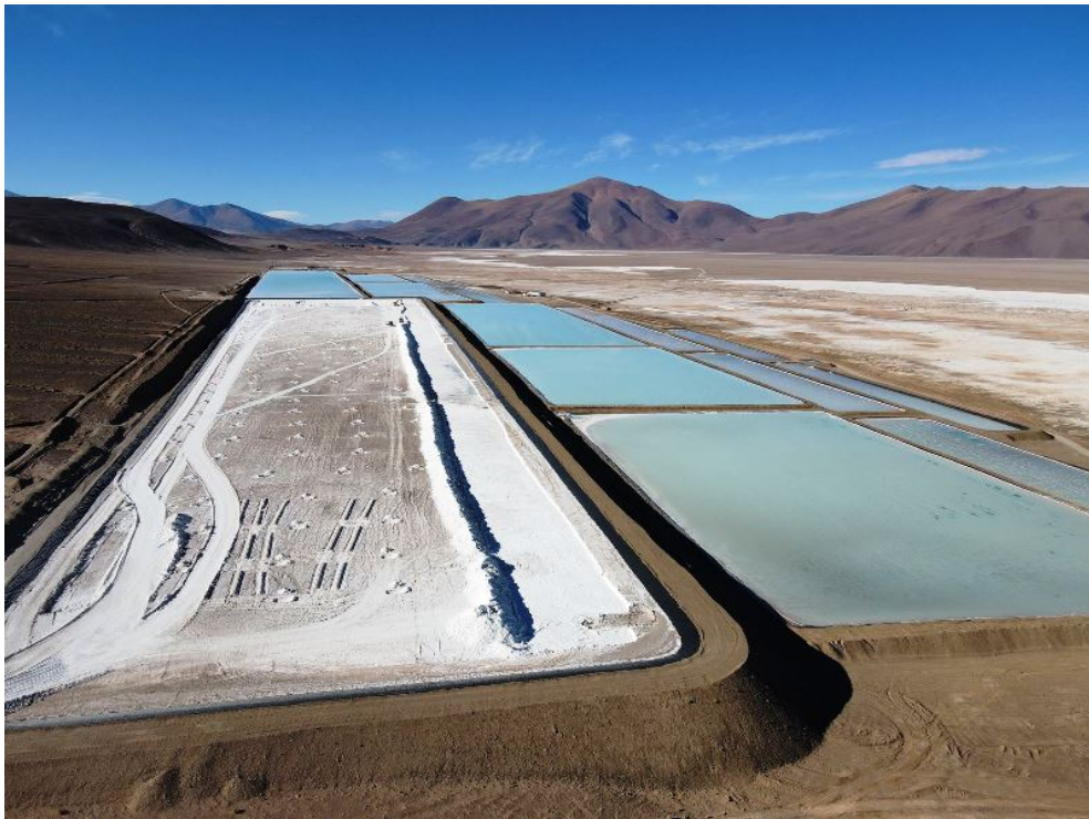
Figure 1. Rincon Lithium Project – Salt Harvesting Works
