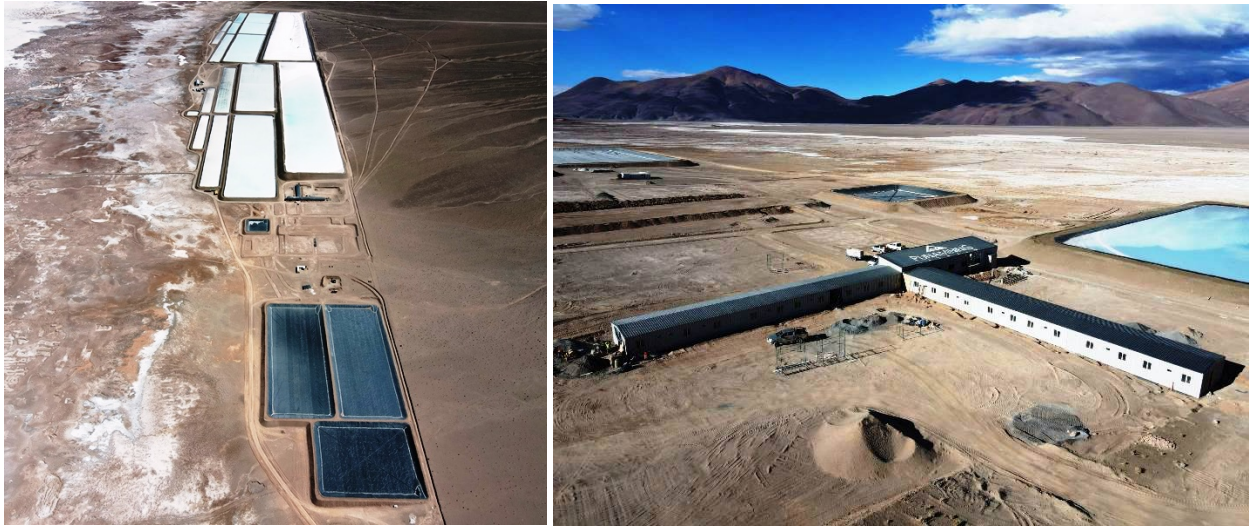
Figures 2-3. Rincon Lithium Project – 2,000tpa Operation Site Works in Progress
