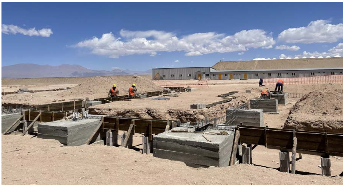
Figure 5. Rincon Lithium Project – 2,000tpa Operation Site Works (industrial plant constructions works)
