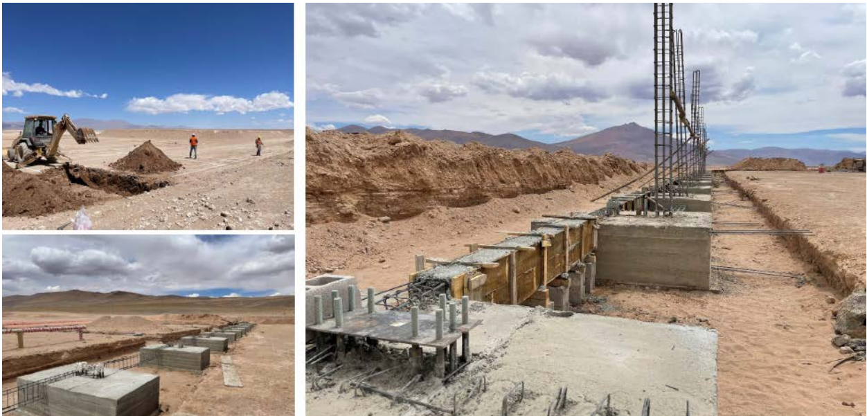
Figure 3. Rincon Lithium Project – 2,000tpa Operation Site Works (industrial plant constructions works)
