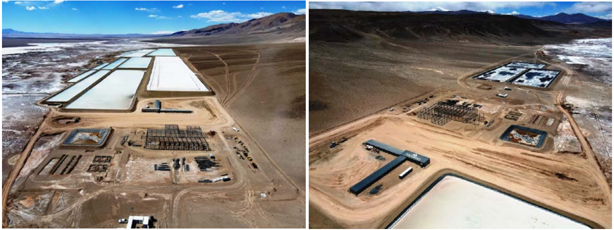
Figures 3-4. Rincon Lithium Project – 2,000tpa Operation Site Works
