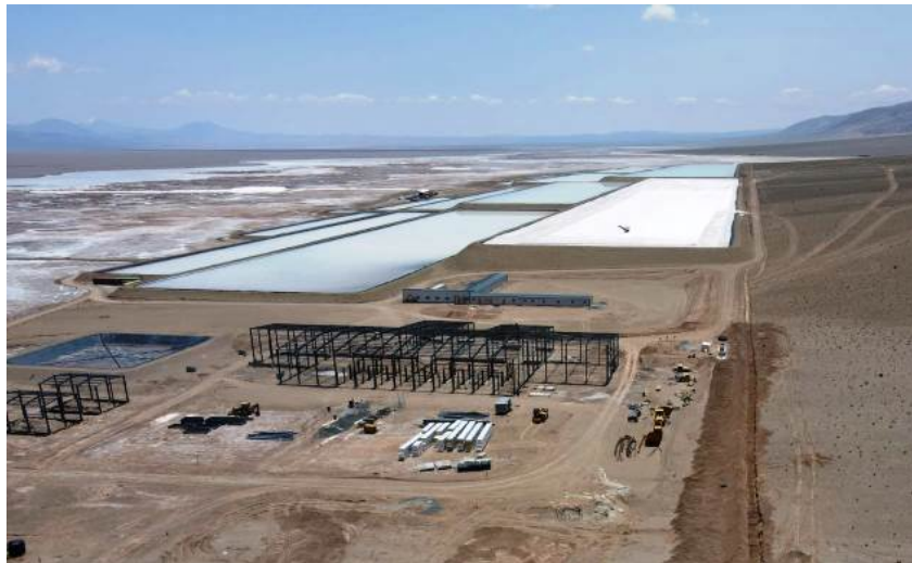
Figure 5. Rincon Lithium Project – 2,000tpa Operation Site Works
