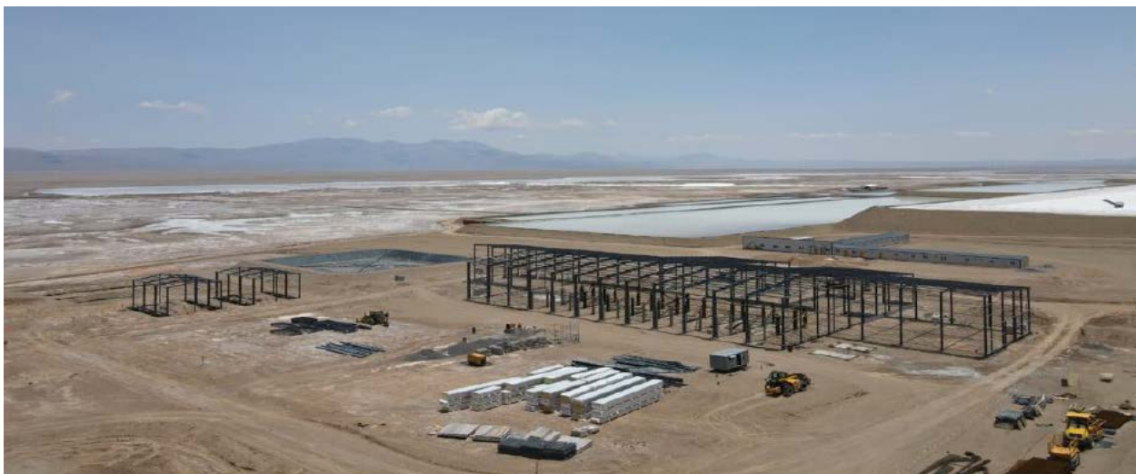
Figure 2. Rincon Lithium Project – 2,000tpa Operation Site Works
