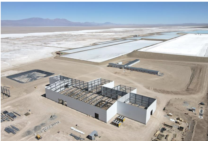
Figure 2. Rincon Lithium Project – 2,000tpa Operation Site Works
