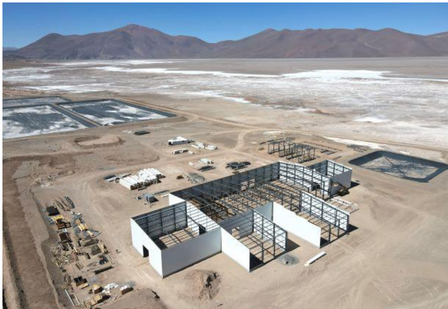
Figure 6. Rincon Lithium Project – 2,000tpa Operation Site Works
