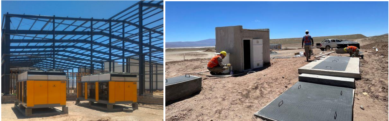
Figures 3-4. Rincon Lithium Project – 2,000tpa Operation Site Works
