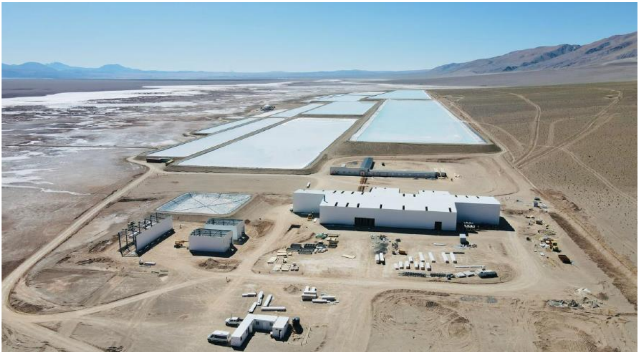
Figure 2. Rincon Lithium Project – 2,000tpa Operation Site Works
