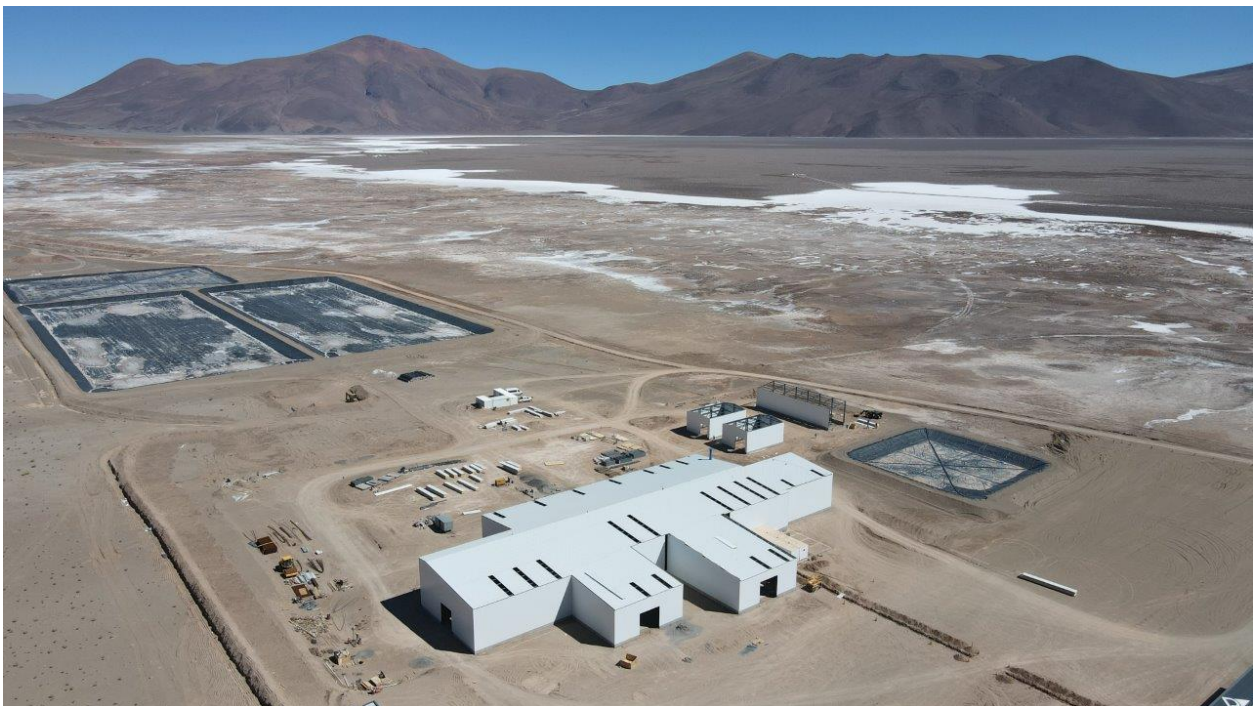
Figure 6. Rincon Lithium Project – 2,000tpa Operation Site Works
