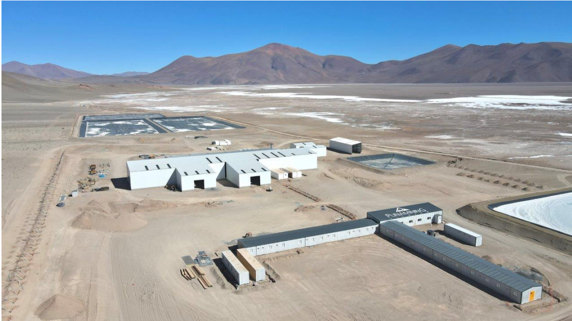
Figure 2. Rincon Lithium Project – 2,000tpa Operation Site Works
