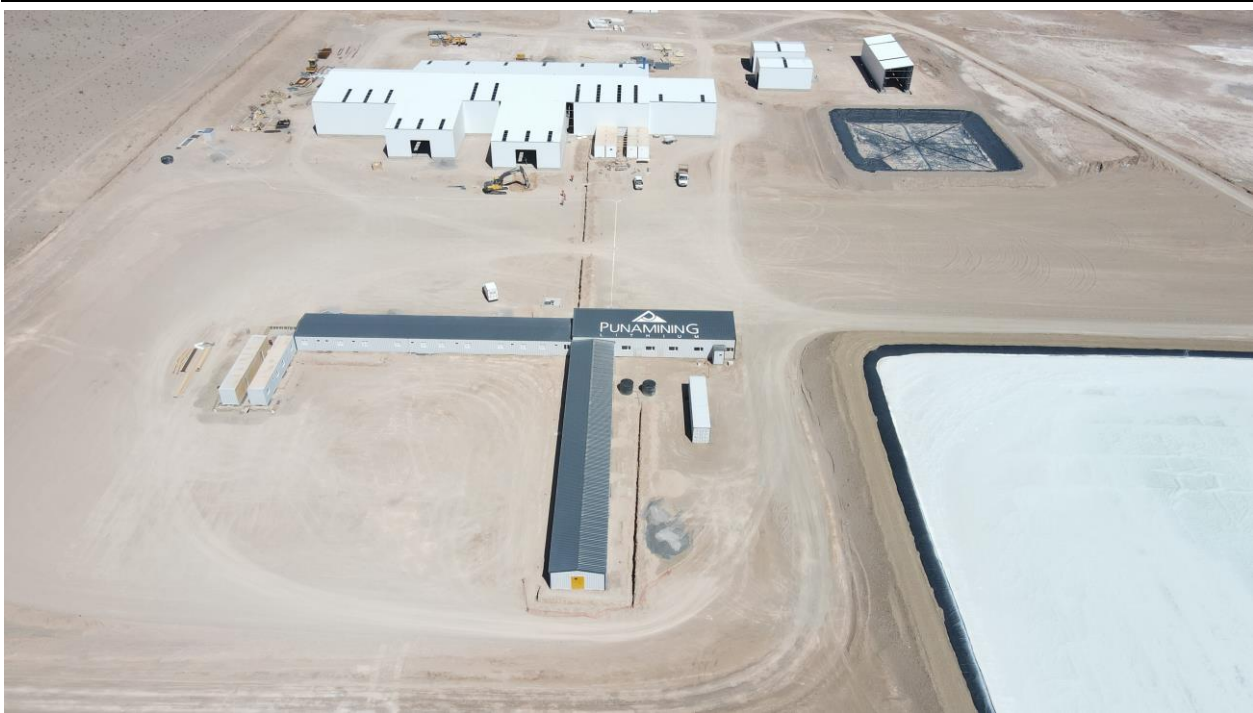
Figure 5. Rincon Lithium Project – 2,000tpa Operation Site Works
