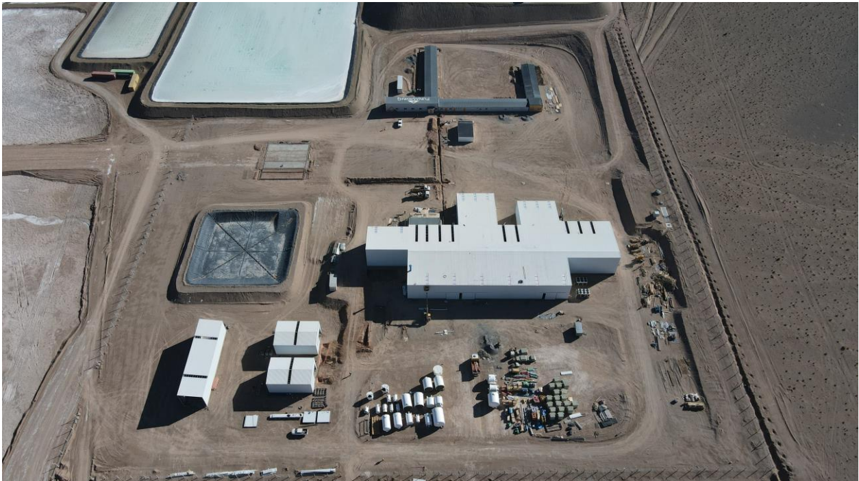
Figure 1. Rincon Lithium Project – 2,000tpa Operation Site Works
