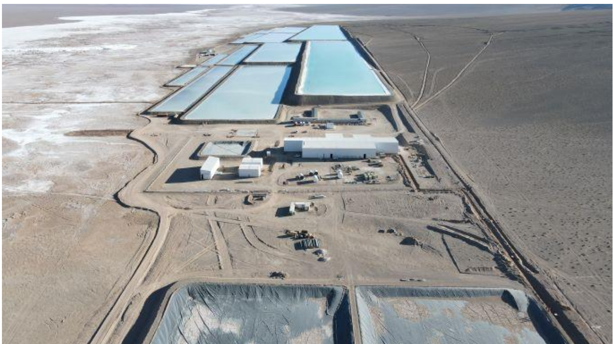
Figure 6. Rincon Lithium Project – 2,000tpa Operation Site Works
