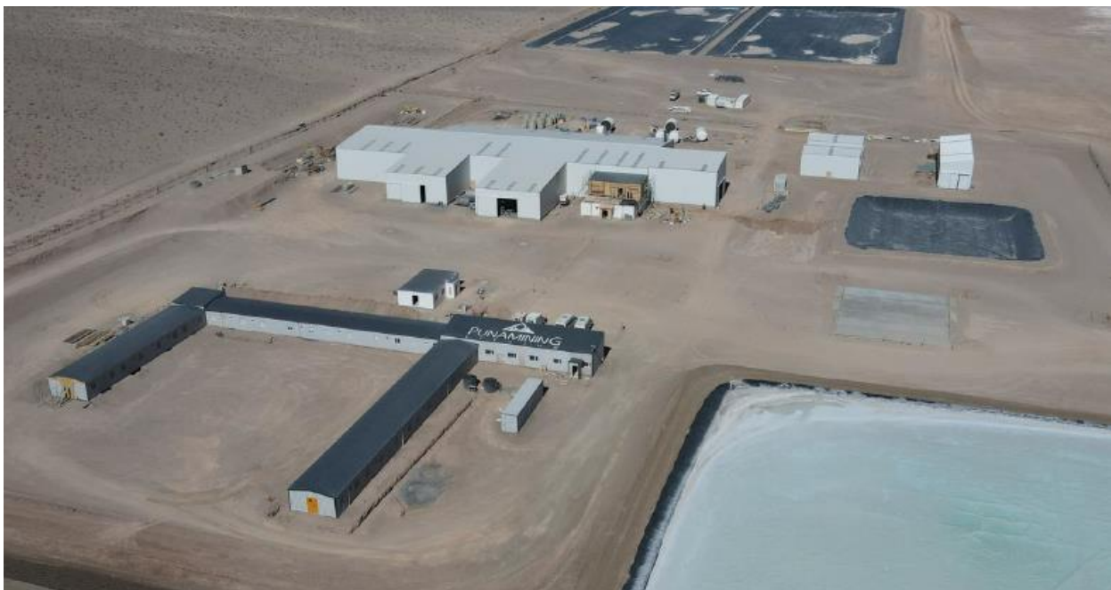
Figure 1. Rincon Lithium Project – 2,000tpa Operation Site Works
