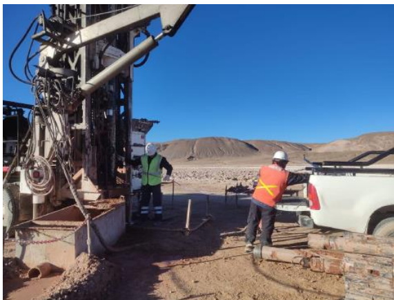
Figures 1-2. Rincon Lithium Project – Production Well Rotary Drilling Works
