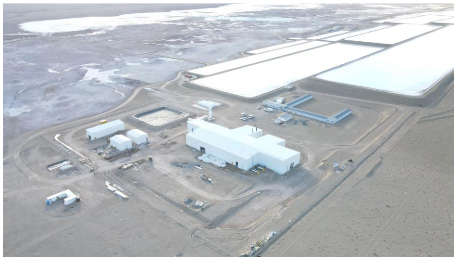
Figure 8. Rincon Lithium Project – 2,000tpa Operations Site
