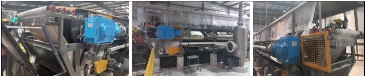
Figures 3-5. Rincon Lithium Project – 2,000tpa Operation Commissioning Works
