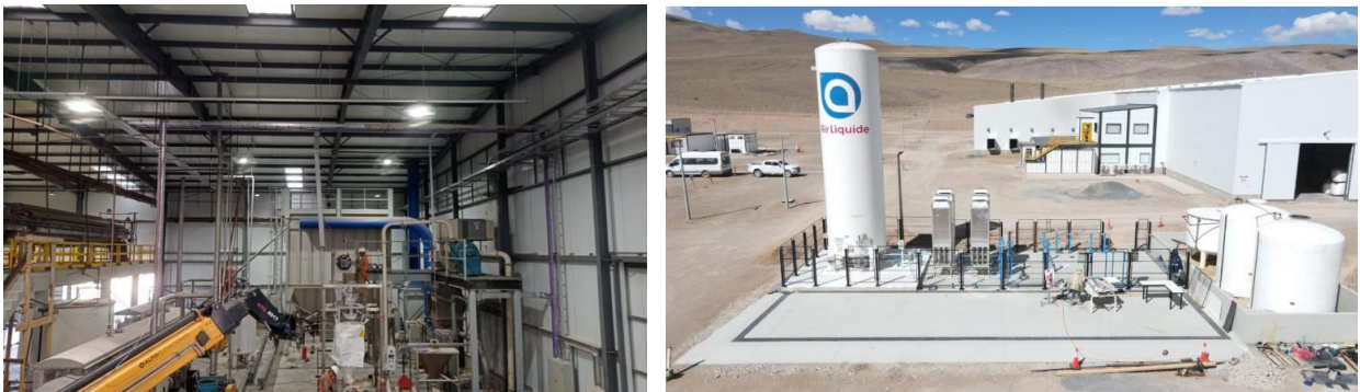
Figures 6-7. Rincon Lithium Project – 2,000tpa Operation Commissioning Works
