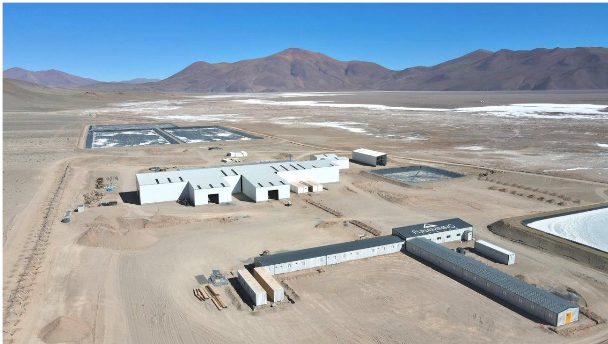
Figure 1. Rincon Lithium Project – 2,000tpa Operation Site Works in Progress
