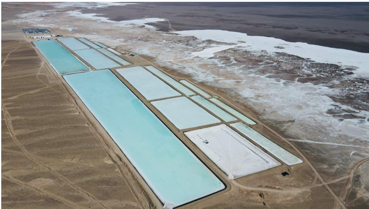
Figure 2. Rincon Lithium Project – 2,000tpa Operation Site Works in Progress
