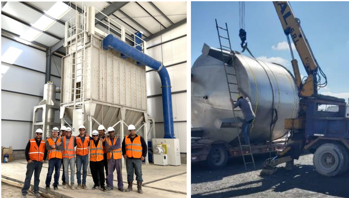
Figures 3-4. Rincon Lithium Project – Operational Equipment Delivered, Installed & Commissioned
