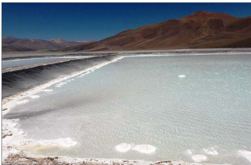
Photos 1 & 2. Rincon Lithium Project – Exploration drilling core and Stage 1 evaporation ponds concentrating lithium brine.
