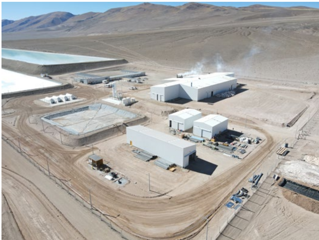
Figure 1. Rincon Lithium Project – 2,000tpa Operations
