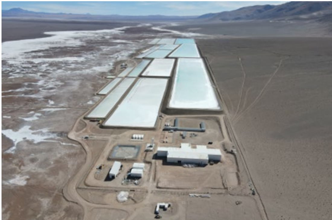
Figure 4. Rincon Lithium Project – 2,000tpa Operations
